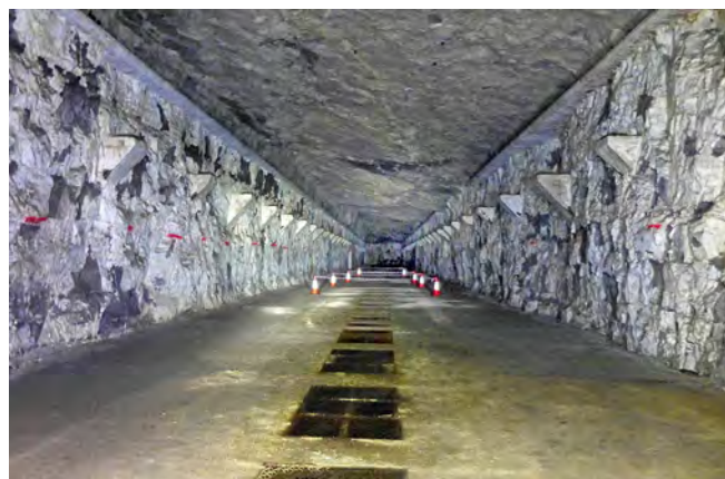
Looking north along storage chamber 'A' from the junction with the main passage. Turning left at the far end leads to the north ventilation shafts. Bollards mark hazards
